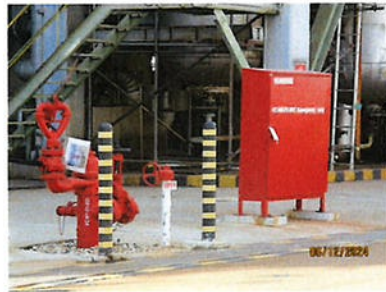
Hydrant with Monitor
